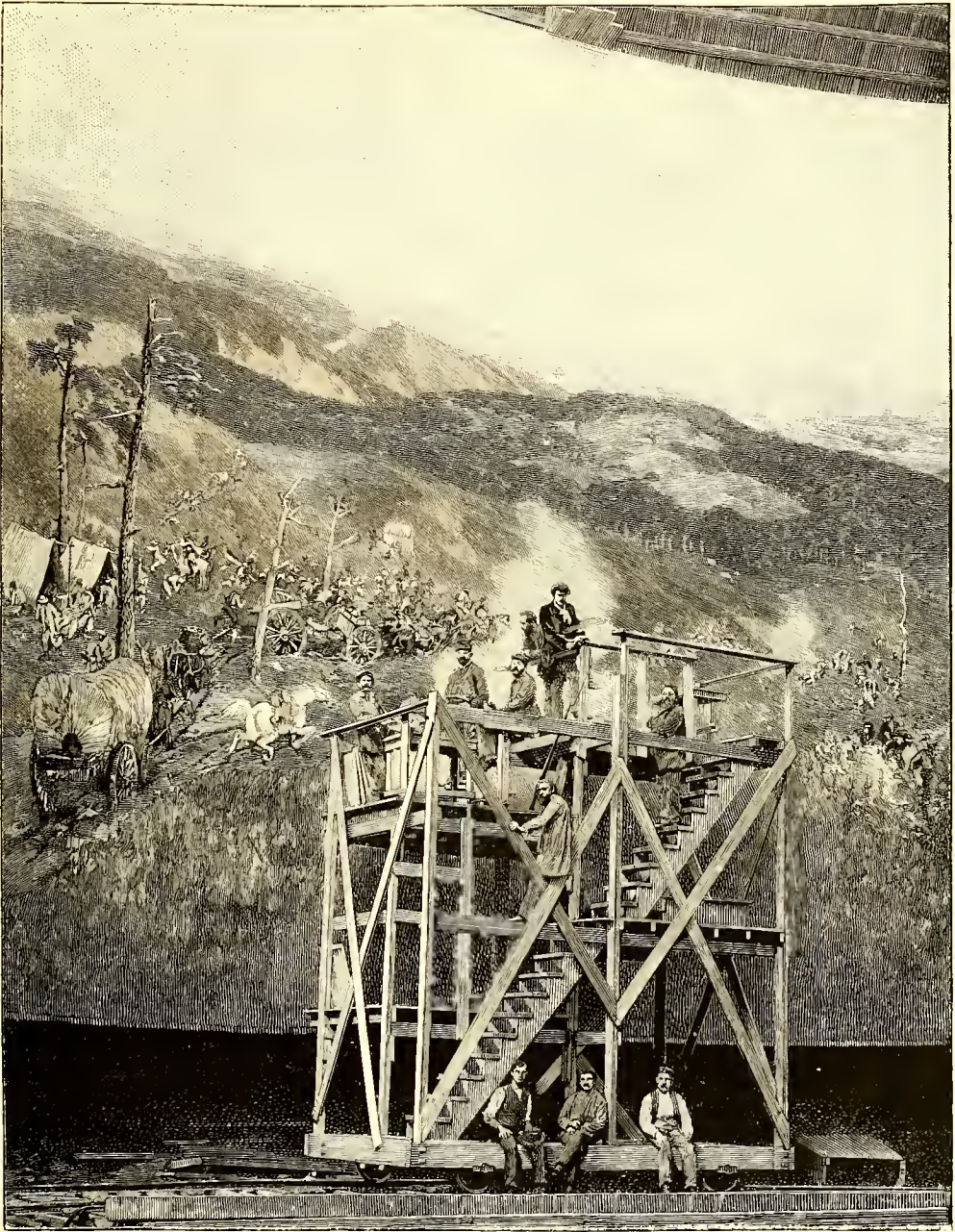
ONE OF THE MOVABLE PLATFORMS USED IN PAINTING A PANORAMA.
